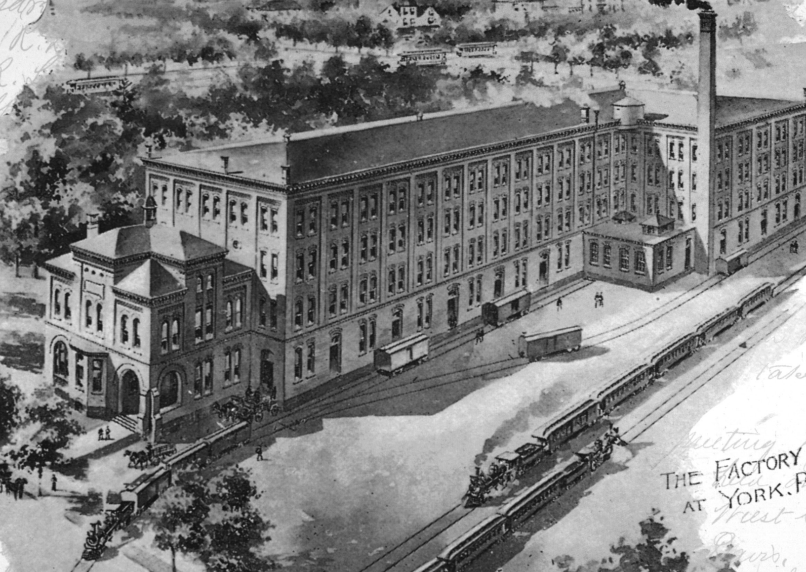
York Wallcoverings Factory 1900s
